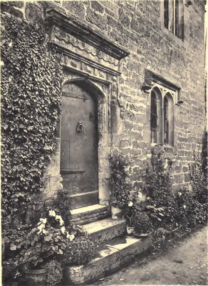
DOORWAY AT WARREN HOUSE, STANTON, GLOS.
