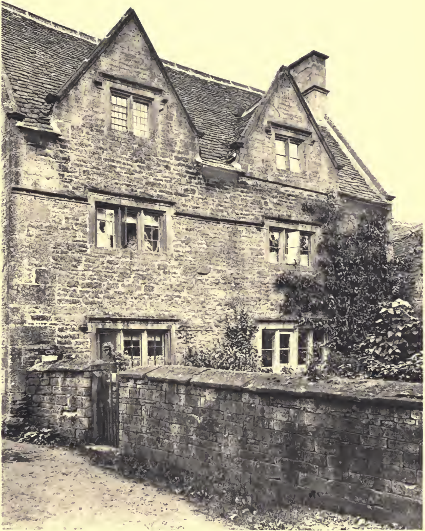
A HOUSE AT BOURTON-ON-THE-WATER, GLOS.
