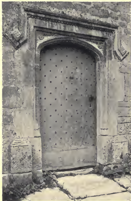
FIG. 15. DOORWAY AT BROADWAY, WORC.
