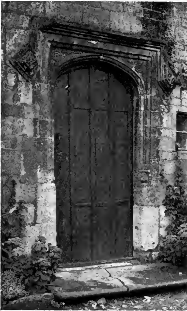
FIG. 14. DOORWAY AT ASTON SUBEDGE.
