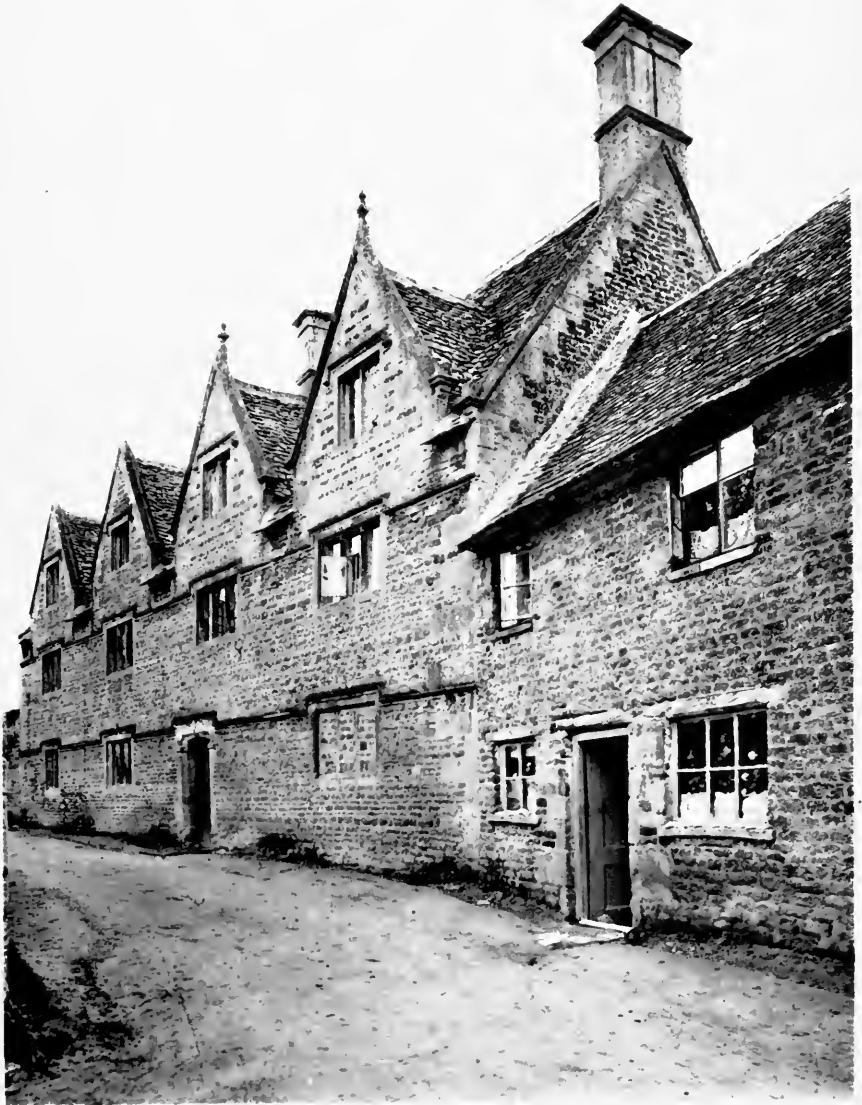
STREET FRONT OF A FARMHOUSE, LITTLE RISSINGTON, GLOS.
