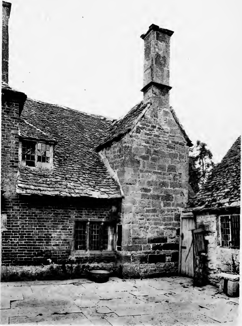
THE KITCHEN CHIMNEY, MEDFORD HOUSE, MICKLETON, GLOS.
