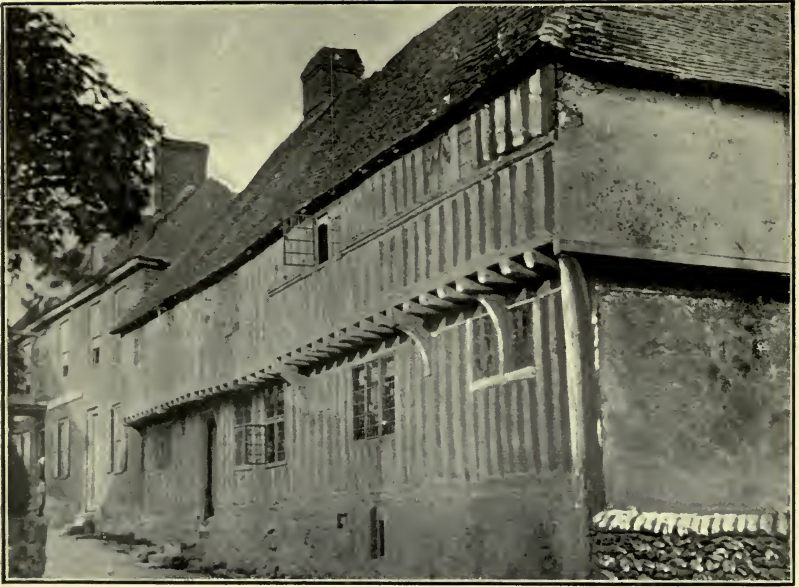
OLD HOUSE, HOLLINGBOURNE
