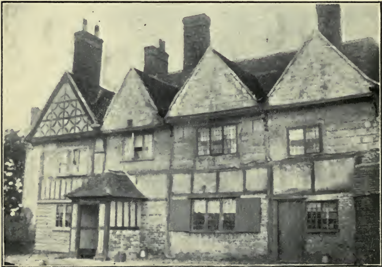
OLD HOUSE NEAR TEYNHAM
