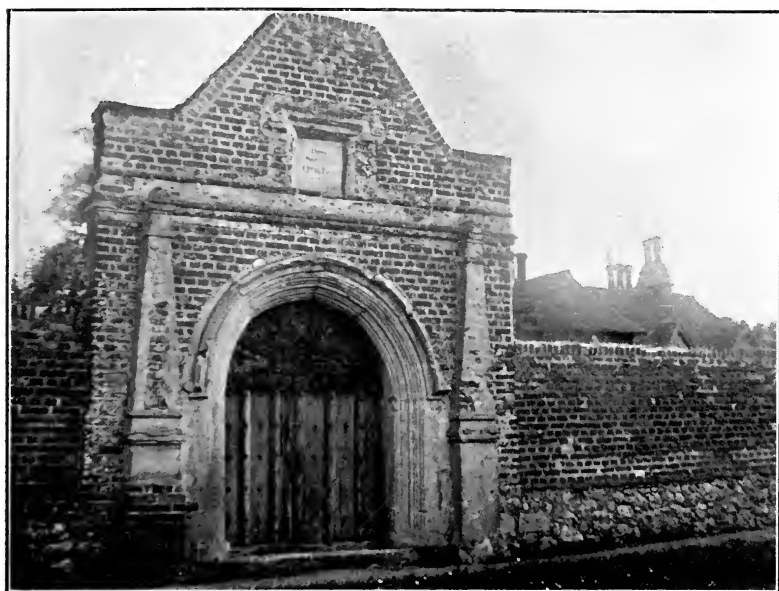
GATEWAY, DAVINGTON COURT
