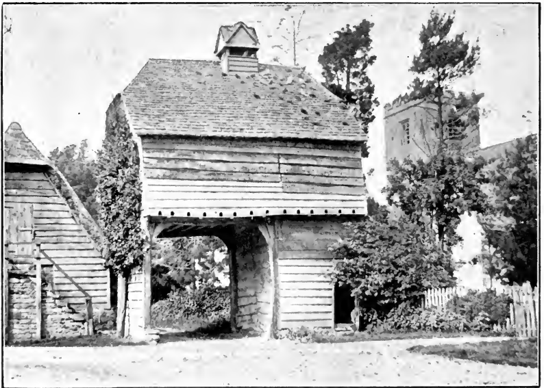
OLD DOVECOTE, NORTHMOOR
