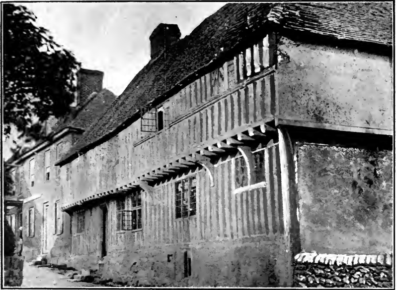
OLD HOUSE, HOLLINGBOURNE
