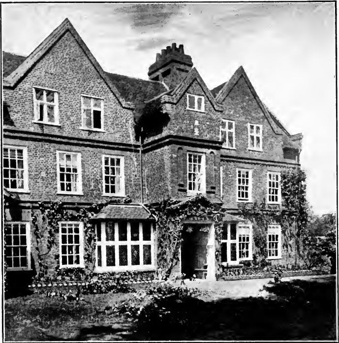
CEDAR HOUSE, HILLINGDON
