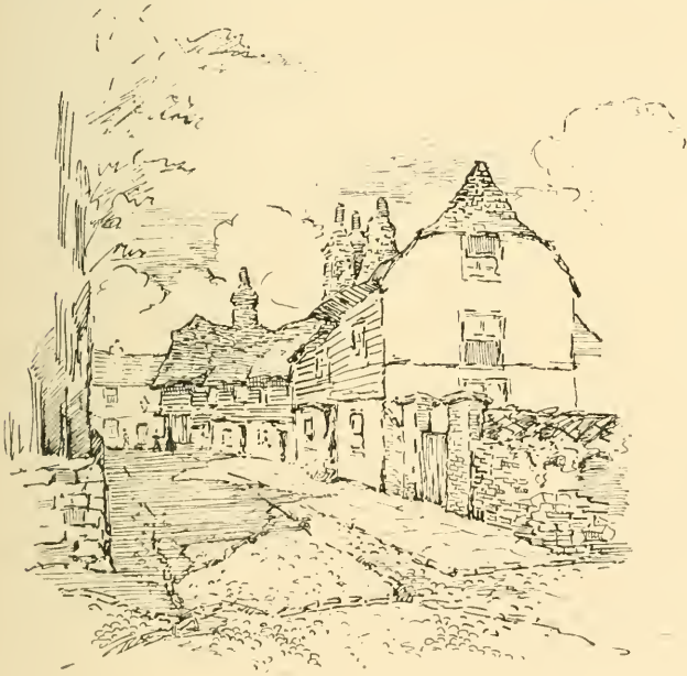
PUMP STREET, RYE.
