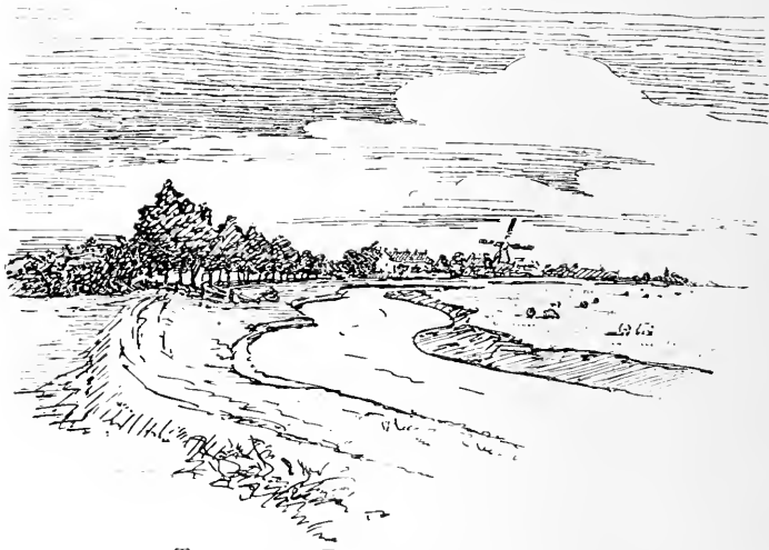
TILLINGHAM RIVER AND WALL, RYE.
