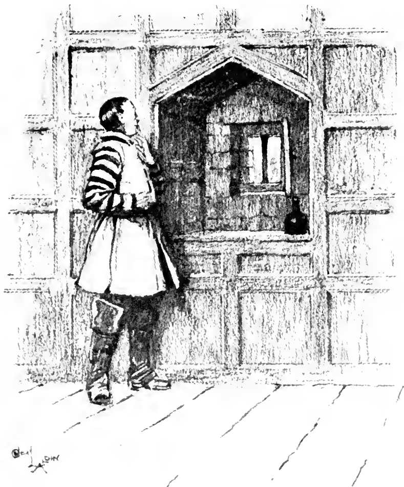
A PEEPHOLE FROM THE SOLAR CHAMBER TO THE GREAT HALL.
