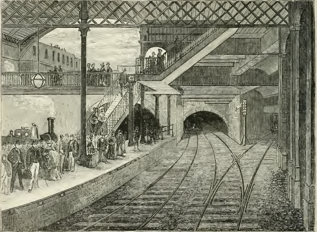
KING'S CROSS UNDERGROUND STATION IN 1868. (See page 227.)
