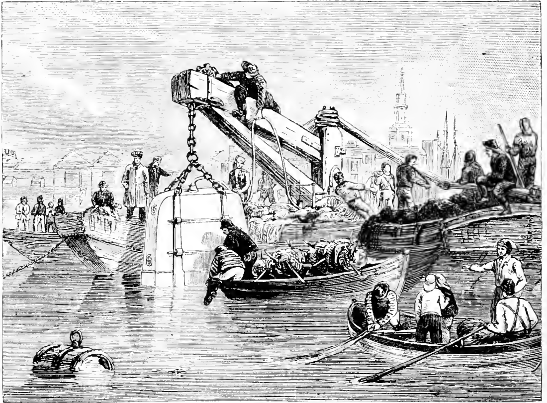
DIVING-BELL USED IN THE CONSTRUCTION OF THE THAMES TUNNEL.
