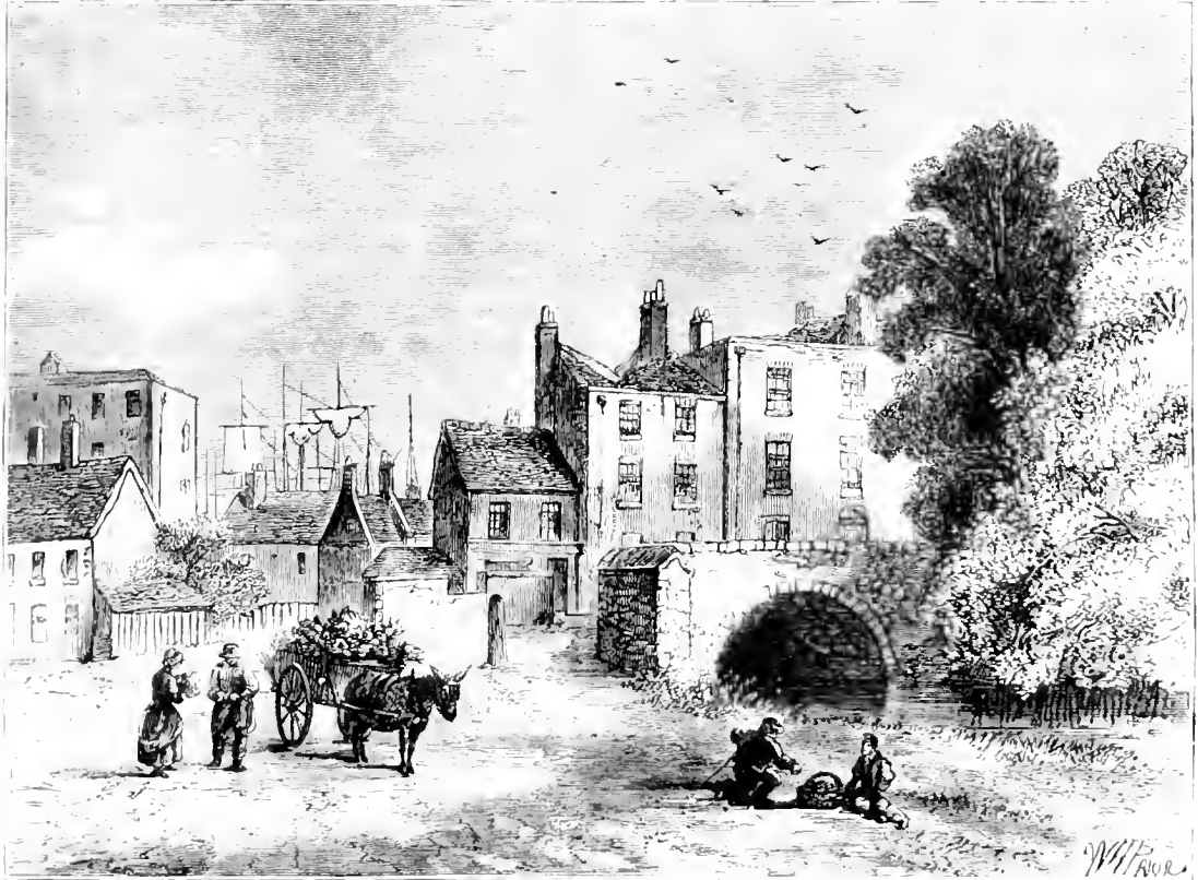
MILL POND BRIDGE, IN 1826.
