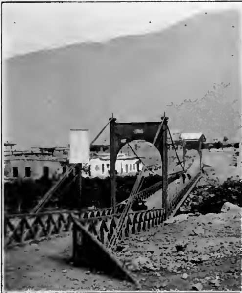
CHOSICA BRIDGE, OROYA ROUTE.
