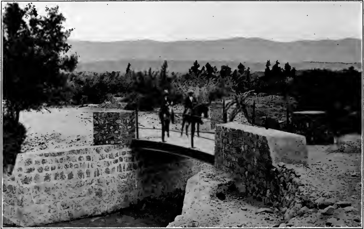
BRIDGE ACROSS THE SAMA RIVER, PROVISIONAL BOUNDARY BETWEEN PERU AND CHILE.
