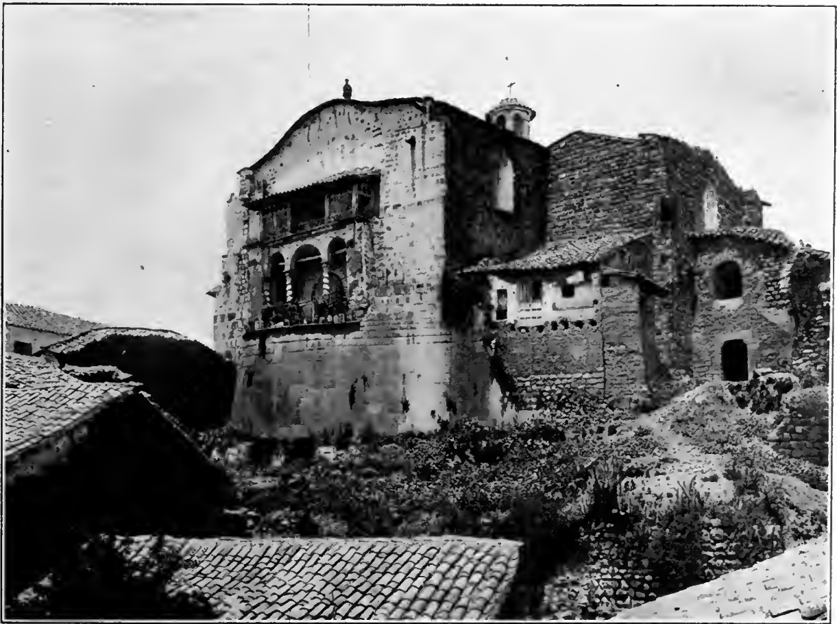
CONVENT OF SANTO DOMINGO, CUZCO, BUILT ON THE FOUNDATIONS OF THE TEMPLE OF THE SUN.
