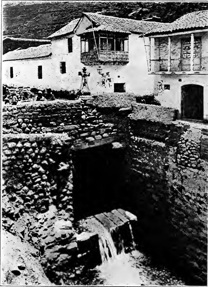
ANCIENT BRIDGE OF SANTA TERESA, CUZCO.
