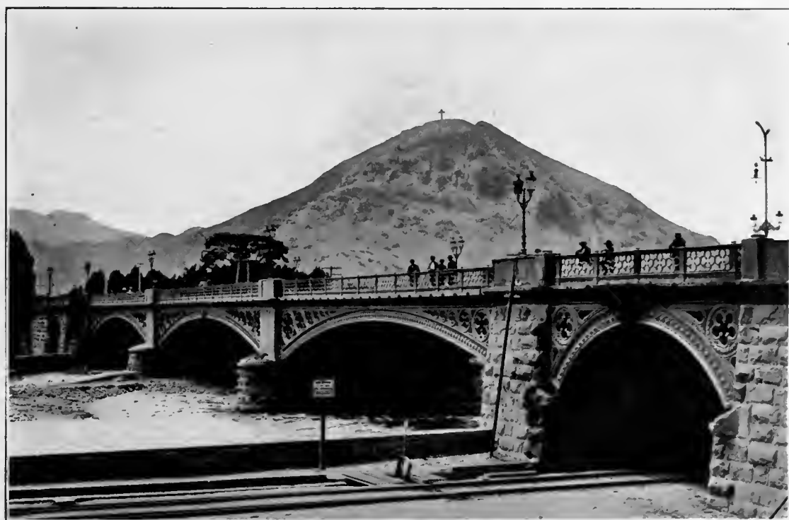
THE BALTA BRIDGE OVER THE RIMAC RIVER.
