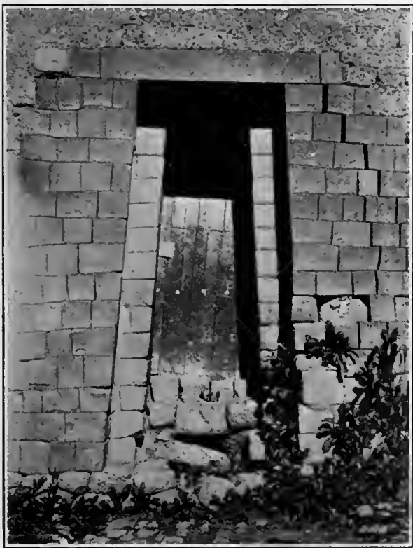
AN INCAIC DOORWAY.
