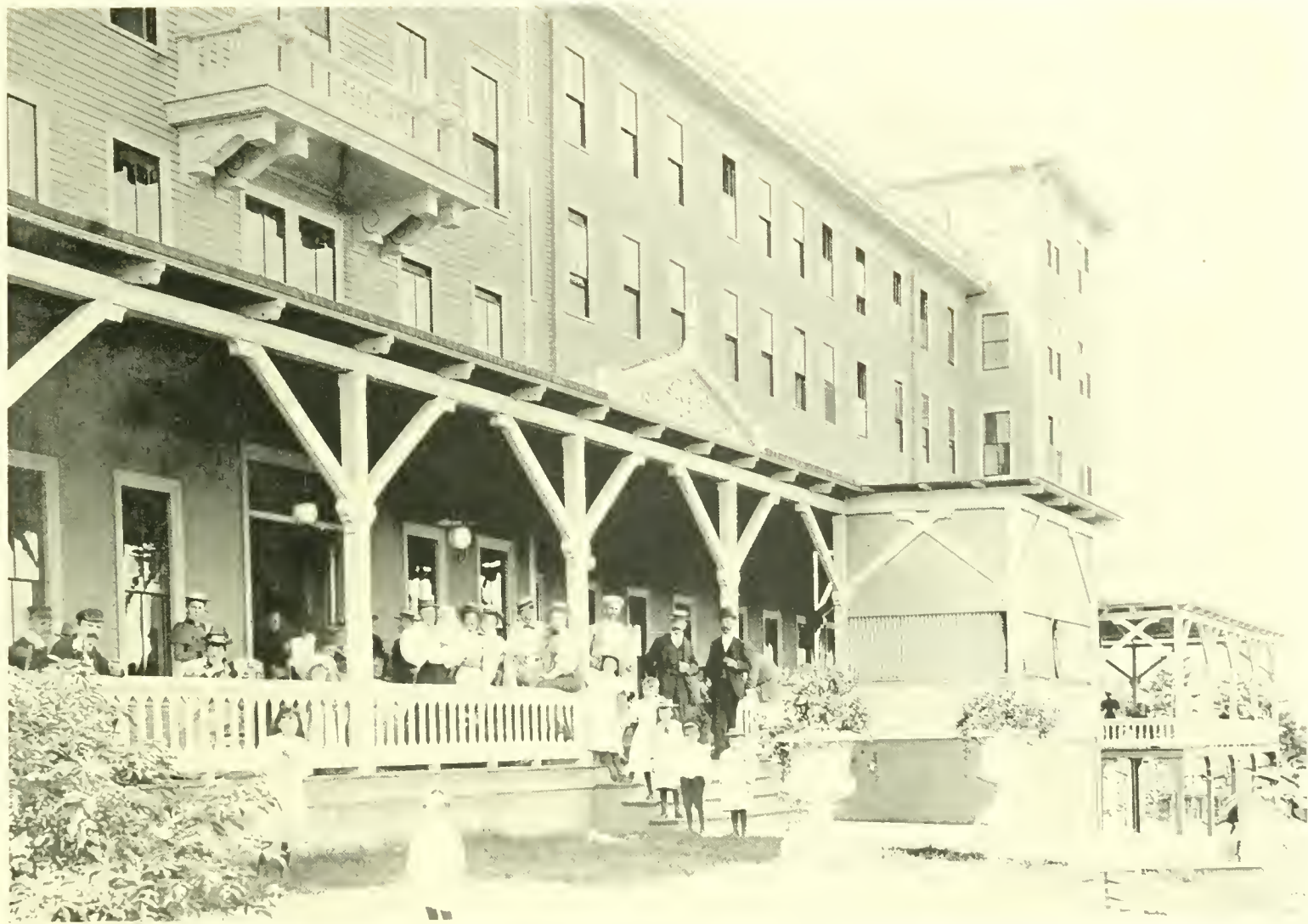
FRONT VIEW OF THE OLD ORCHARD HOUSE.
