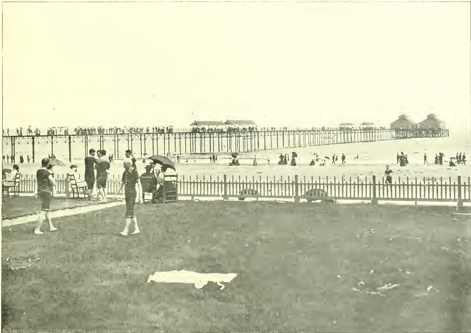
SIDE VIEW OF THE PIER.
