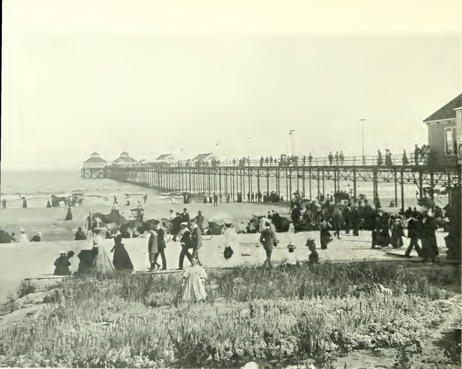
VIEW OF THE STEEL PIER FROM THE SHORE.
