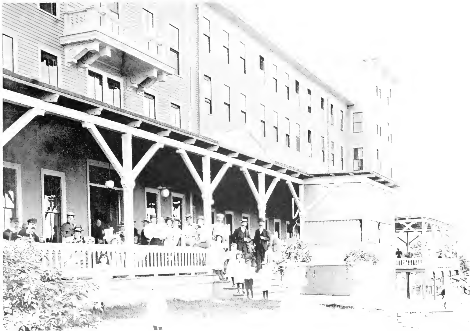
FRONT VIEW OF THE OLD ORCHARD HOUSE
