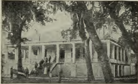
THE MISSISSIPPI BUILDING
