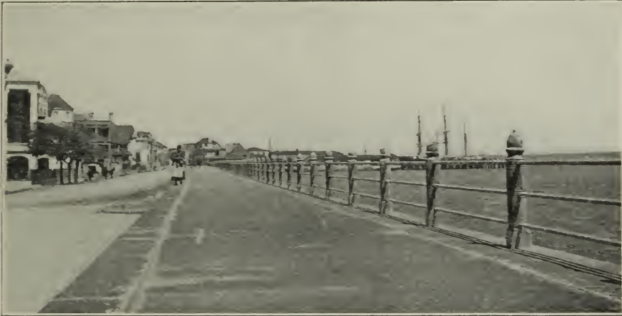
THE BATTERY, CHARLESTON, SOUTH CAROLINA
