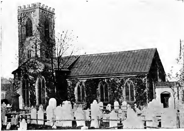
CHRIST CHURCH, UPPER MERION (OLD SWEDES) BRIDGEPORT, PENNSYLVANIA. BUILT BY DR. WRANGEL AND DEDICATED JUNE 25TH, 1760.
