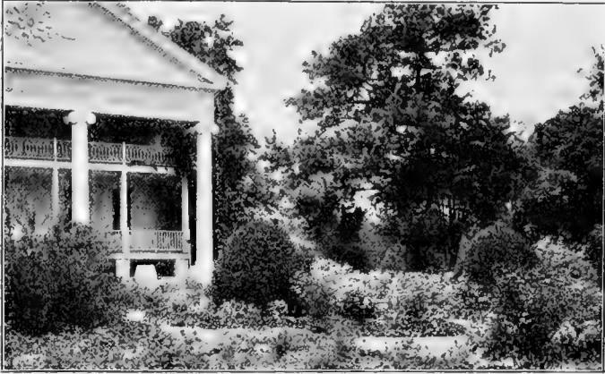
Greenwood, Thomasville, Georgia.
