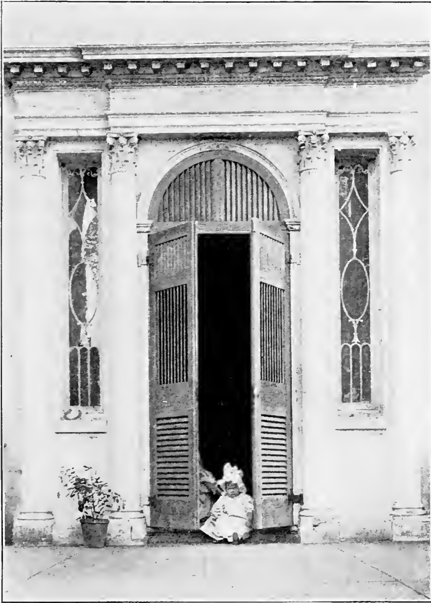
OLD DOORWAY AT OATLANDS
