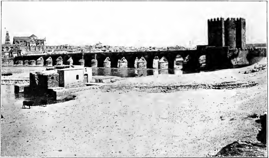
THE OLD BRIDGE AT CORDOVA.
