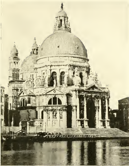
THE EXTERIOR OF SALUTE'S DOME.
