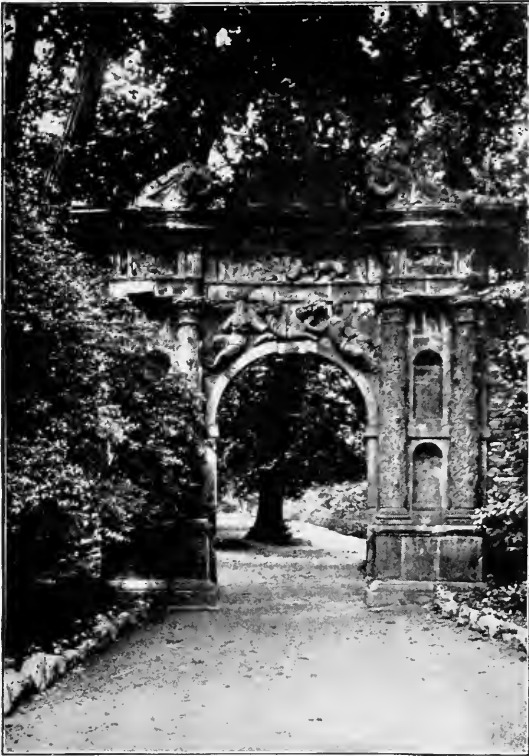
THE ELIZABETH GATE IN THE CASTLE GROUNDS.
