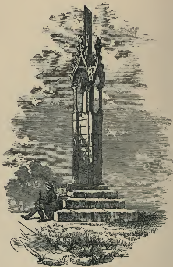
Mill Bridge Cross.
