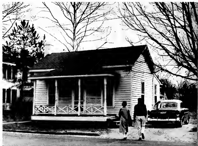
THE OFFICE BUILDING ANNEX
