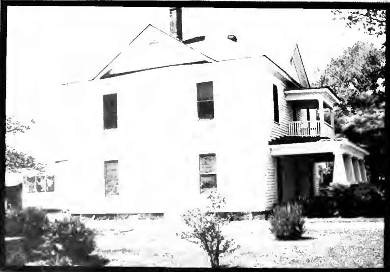
This view of typical dormitory living shows the progress Mount Olive College has seen after all these years.
