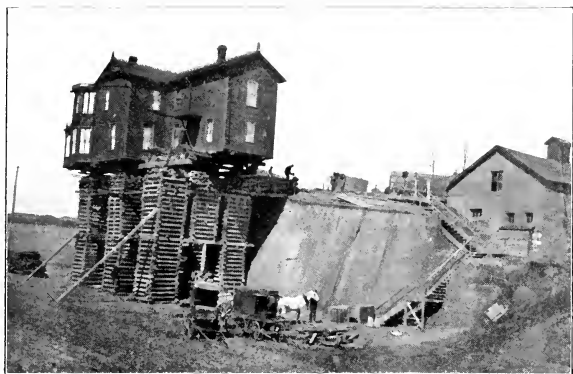
CUTTING DOWN THE DOUGLAS STREET HILL IN THE EARLY '90s The N. B. Falconer House, corner of Nineteenth Street
