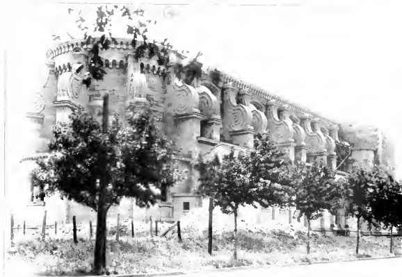
VIEWS OF ST. CECILIA'S CATHEDRAL, OMAHA In course of construction
