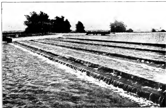
SETTLING BASINS, OMAHA WATER COMPANY, AT FLORENCE
