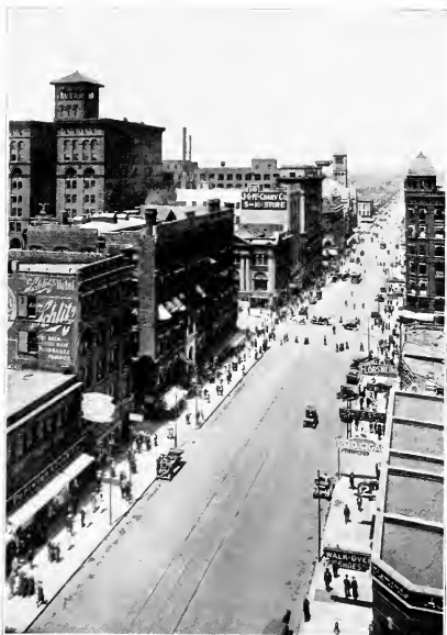
VIEW OF SIXTEENTH STREET FROM HARNEY NORTH, OMAHA
