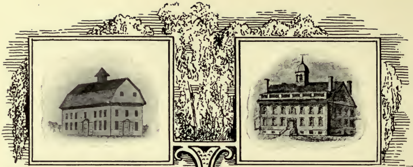
FIRST STATE HOUSE AT HARTFORD COMMENCED IN 1719; OCCUPIED IN 1720 FRAME BUILDING 30 X 70 FEET 24 FEET IN HEIGHT
