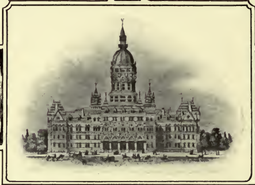
THIRD STATE HOUSE AT HARTFORD COMMENCED IN 1874; OCCUPIED IN 1878; LENGTH 296 FEET. WIDTH, 190 FEET; HEIGHT TO TOP OF ROOF 93 FEET AND TO TOP OF CROWNING FIGURE ON THE DOME 257 FEET.
