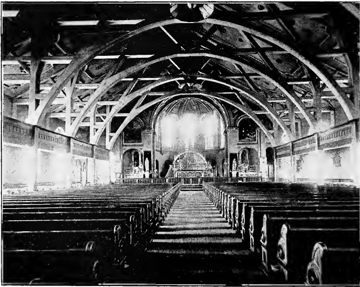
INTERIOR ST. JOSEPH'S CHURCH, LOWELL.
