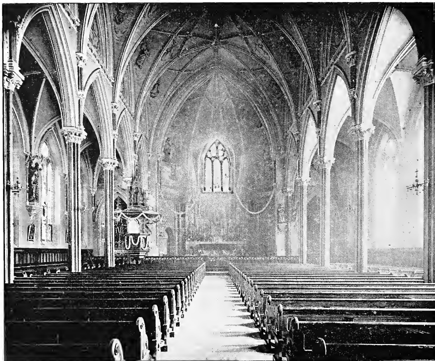
INTERIOR CHURCH OF THE HOLY TRINITY BOSTON.
