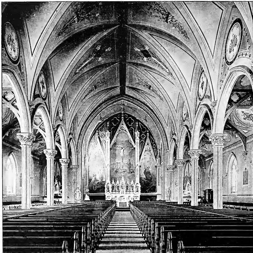
INTERIOR ST. JOHN'S CHURCH, PEABODY.
