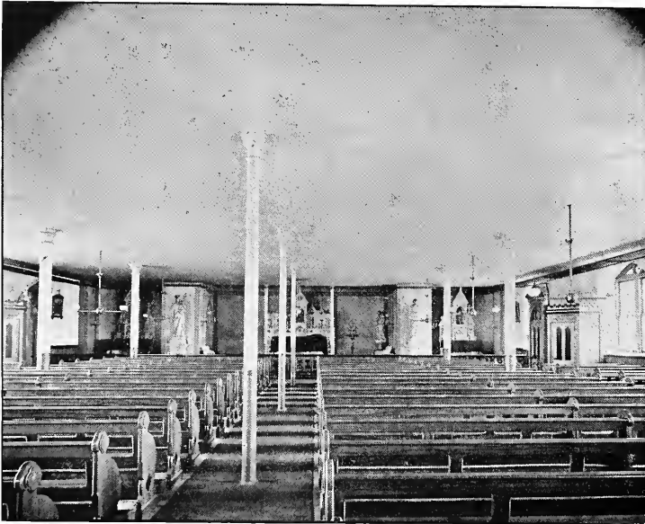
INTERIOR BASEMENT, ST. MARY'S CHURCH, DEDHAM.
