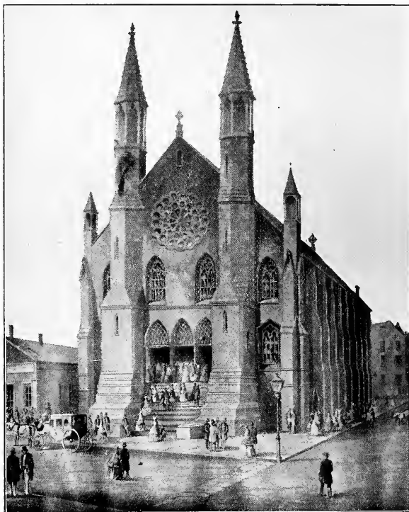
OLD ST. JAMES' CHURCH, ALBANY STREET.
