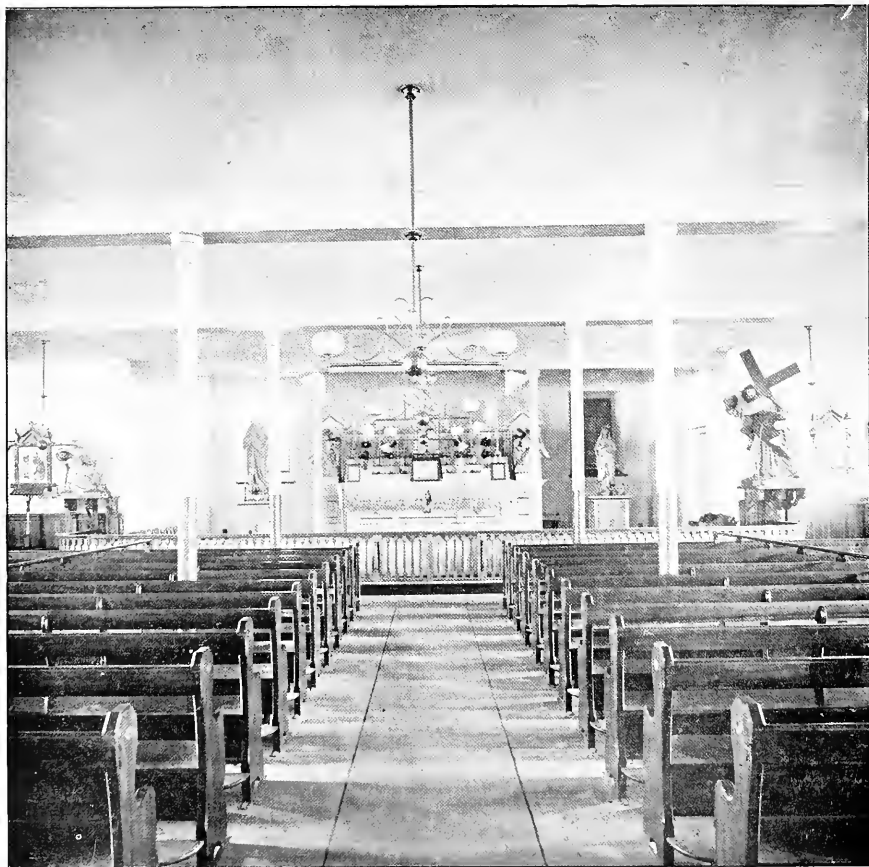
INTERIOR BASEMENT CHURCH OF THE SACRED HEARTS, MALDEN.
