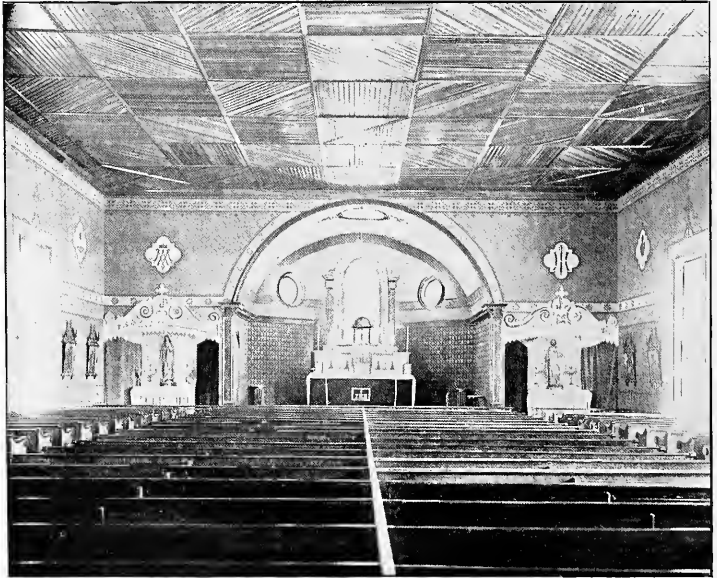
INTERIOR ST. GEORGE'S CHURCH, SAXONVILLE.
