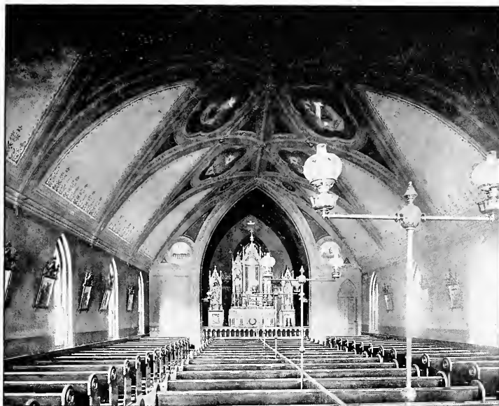
INTERIOR ST. PATRICK'S CHURCH, GROVELAND.
