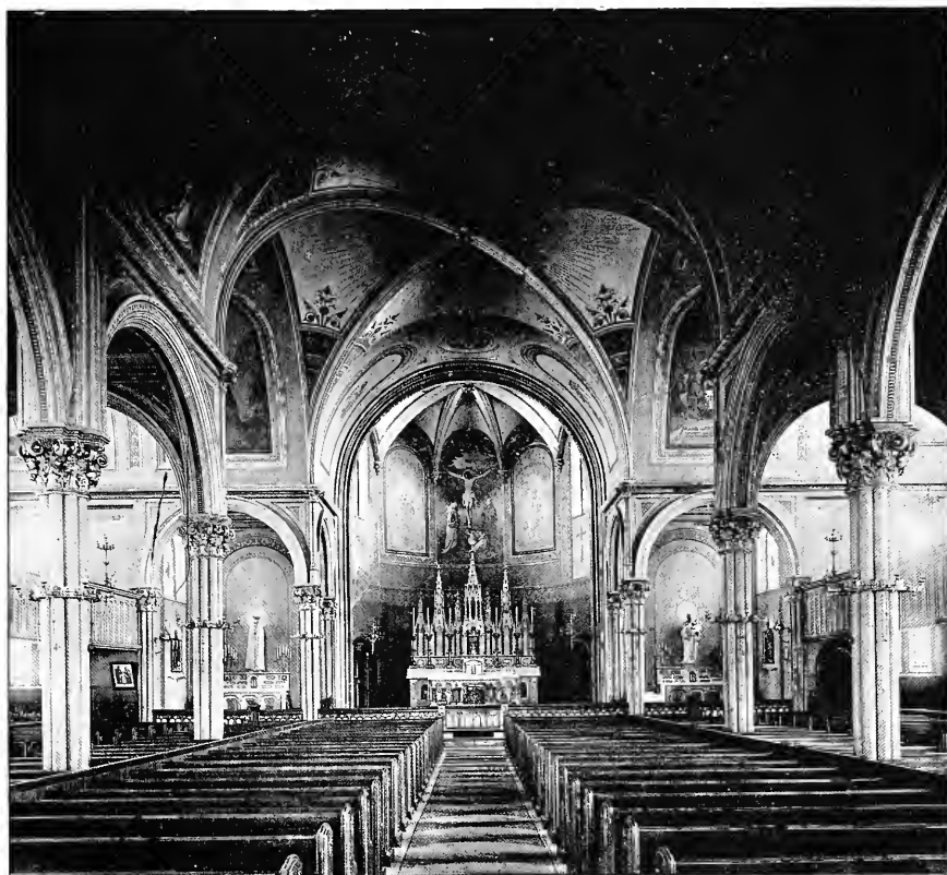
INTERIOR ST. MARY'S CHURCH, WALTHAM.
