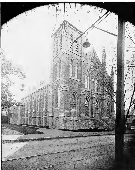
ST. MARY'S CHURCH, DEDHAM.
