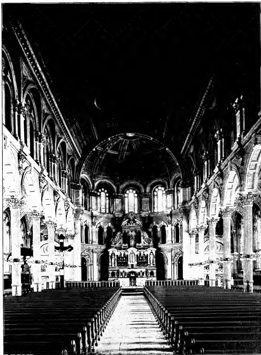
INTERIOR ST. MARY'S CHURCH, BOSTON.
