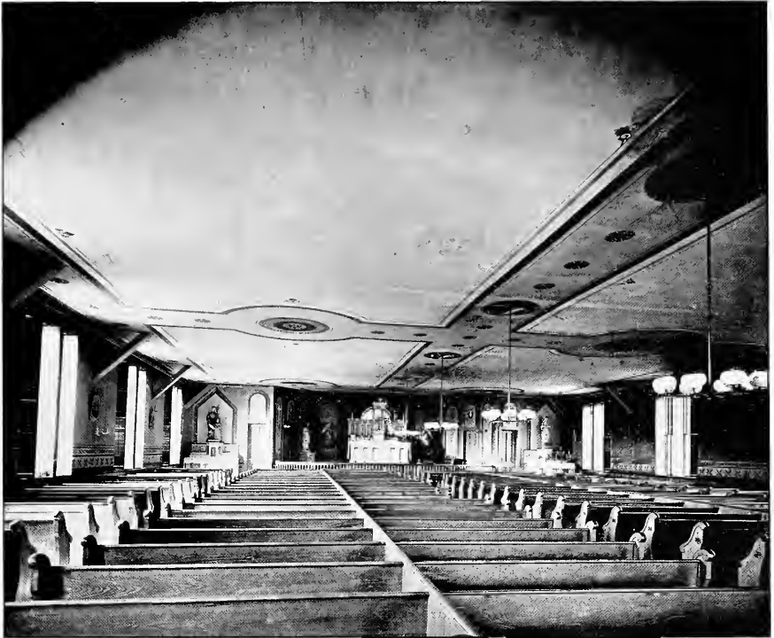
INTERIOR ST. ANNE'S CHURCH, SOMERVILLE.
