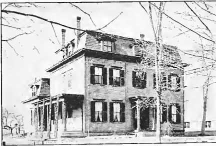
PAROCHIAL RESIDENCE, ST. THOMAS AQUINAS CHURCH, BRIDGEWATER.
