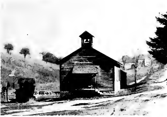
Pine Run School — original building
