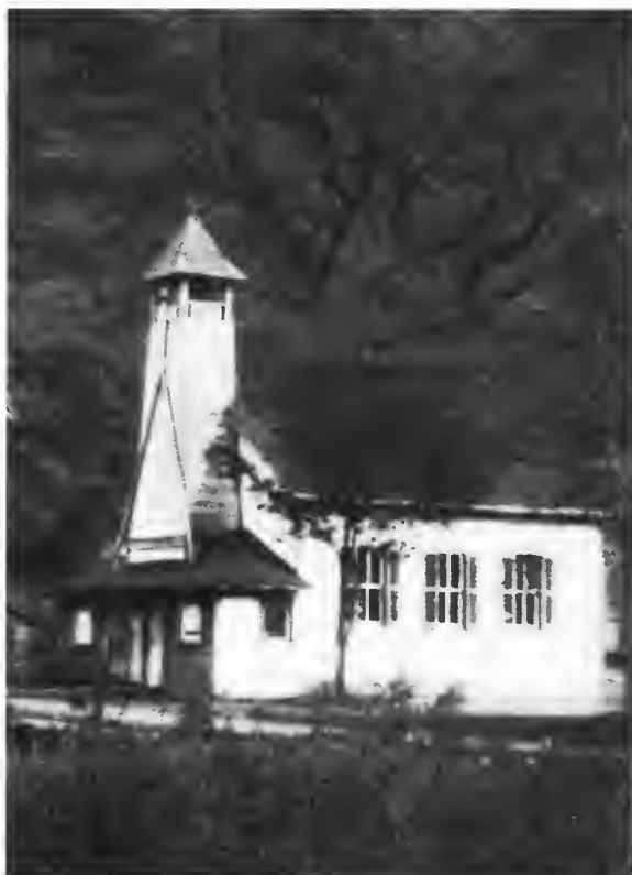
Jersey Mills School — The rooms on either side of the belfry were added as cloak rooms and chemical toilets. The pipe in front is an air vent for the toilets. c.1926
