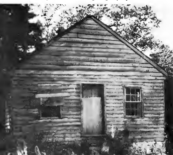
Steuben School — Cogan House Township. 1846-1894. In 1894 a new school was built, and the old log school was covered with weatherboards and used as a blacksmith's shop.
