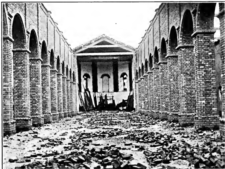
CATHEDRAL IN ERECTION AT NYUNDE
