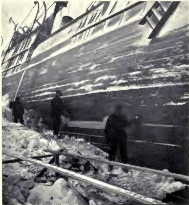
THE LEAK MENDED
