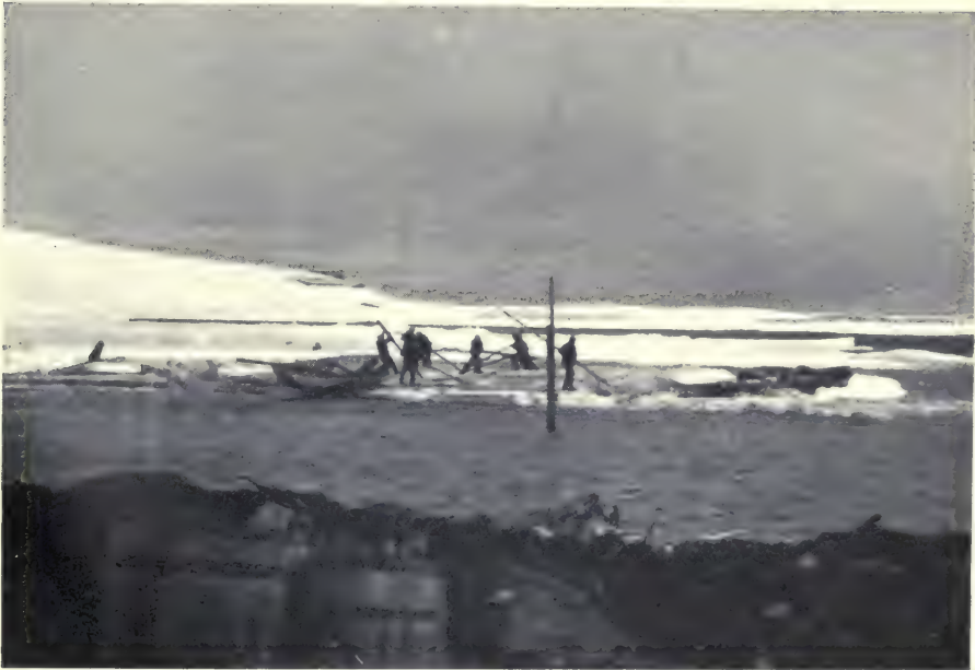
MAKING A CANAL TO LIBERATE THE SHIP
