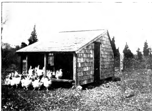
Modern Tolman house of the improved open-front or fresh-air type as used by Joseph Tolman, Rockland, Mass.
