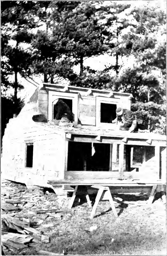
Building a Woods' house, 10x16 ft., portable colony type. Wozelma Farms Producing Co., Silver Lake, Mass. (Photo by John E. Zeller.)
