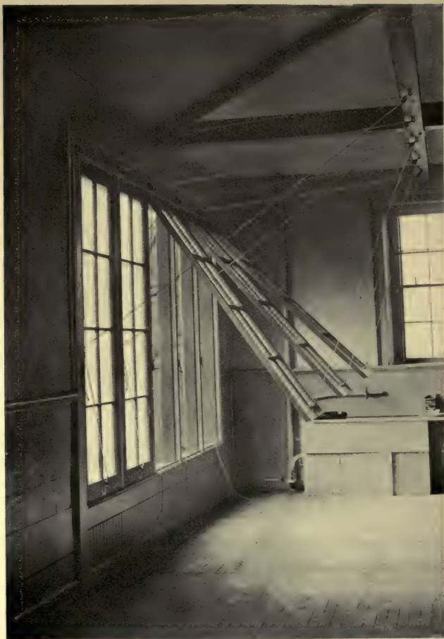
The windows in the Providence school are hinged at the top and can be raised against the ceiling by cords and pulleys
