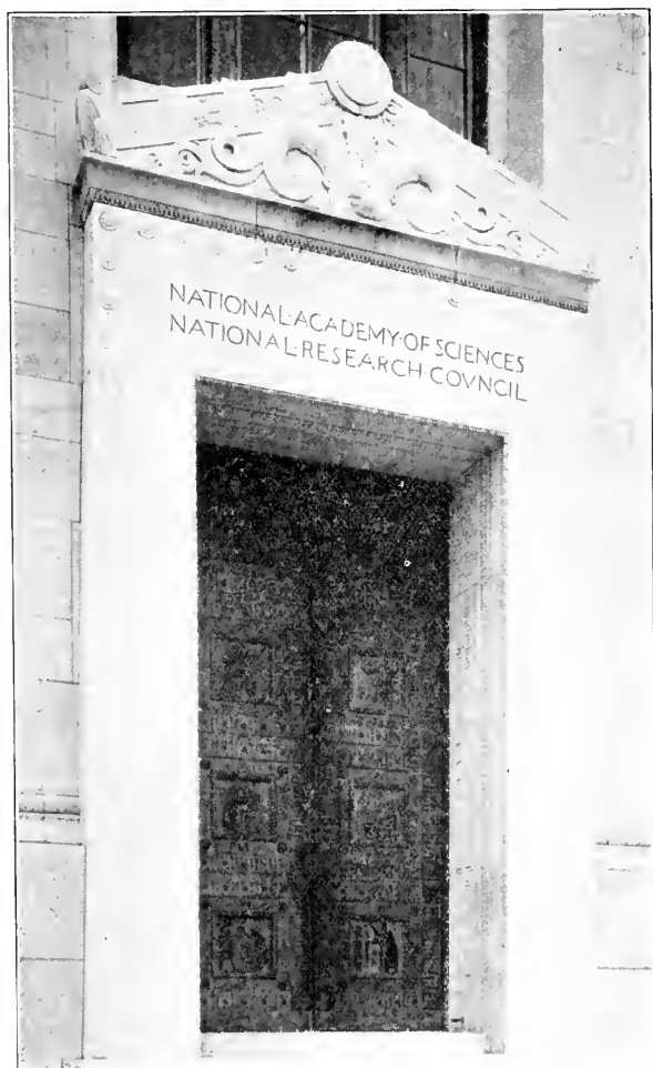
ENTRANCE, SHOWING BRONZE DOORS CLOSED.
