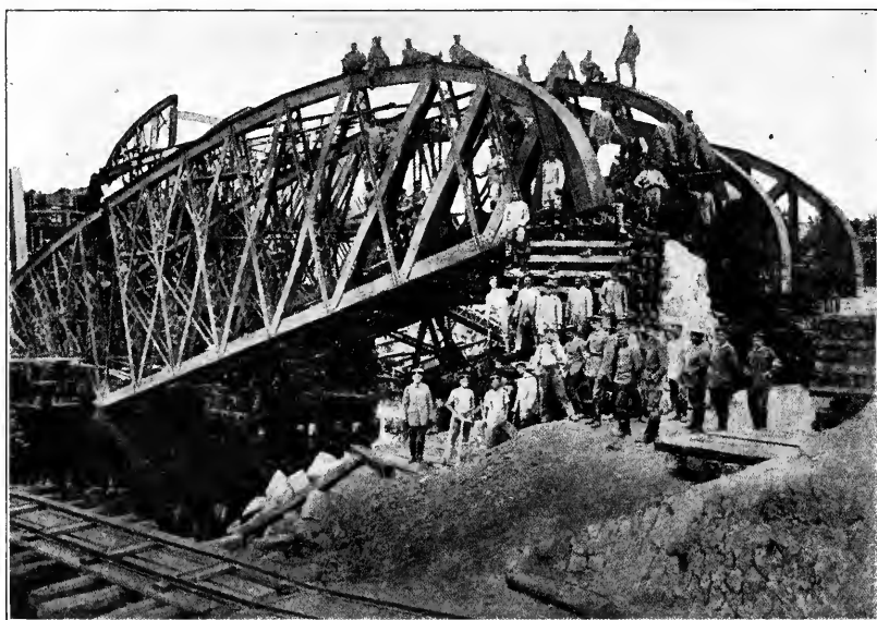
GERMAN PIONEERS RECONSTRUCTING A BRIDGE IN GALICIA.
