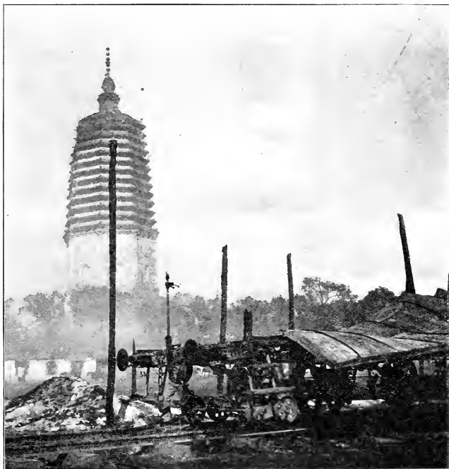
12. HOKU SHAN TOWER.
