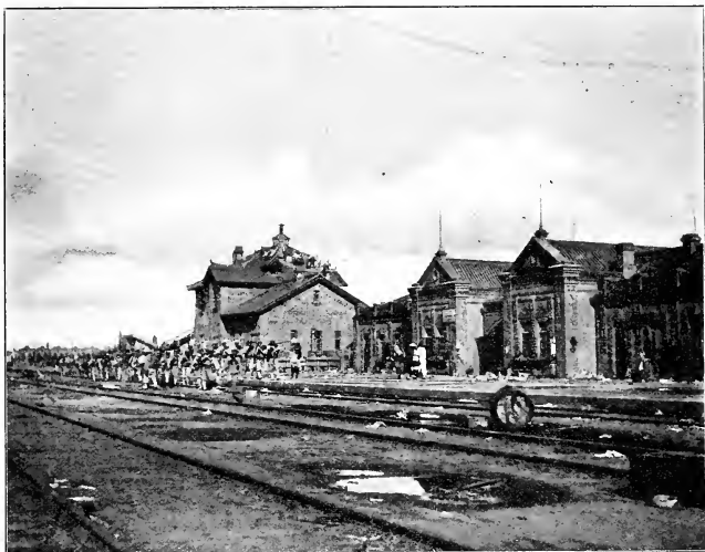
6. TAKING POSSESSION OF THE LIAO YANG RAILWAY STATION.
