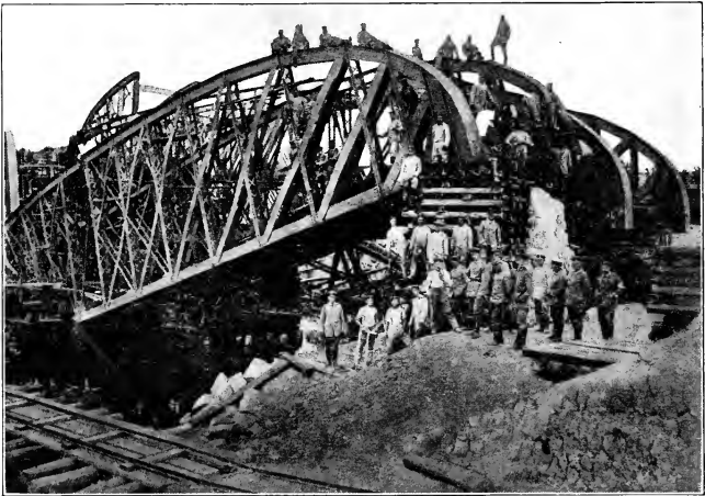
A BRIDGE IN GALICIA BLOWN UP BY THE RETREATING RUSSIANS, BEING INSPECTED BY GERMAN ENGINEERS WITH A VIEW TO RECONSTRUCTION.
