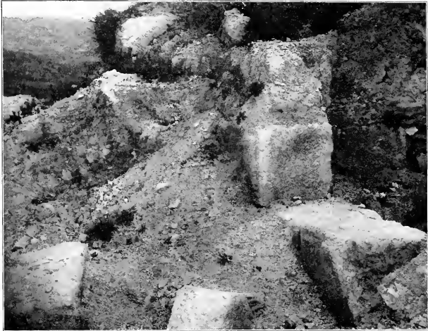
UPPER WALL, LOOKING EAST.
