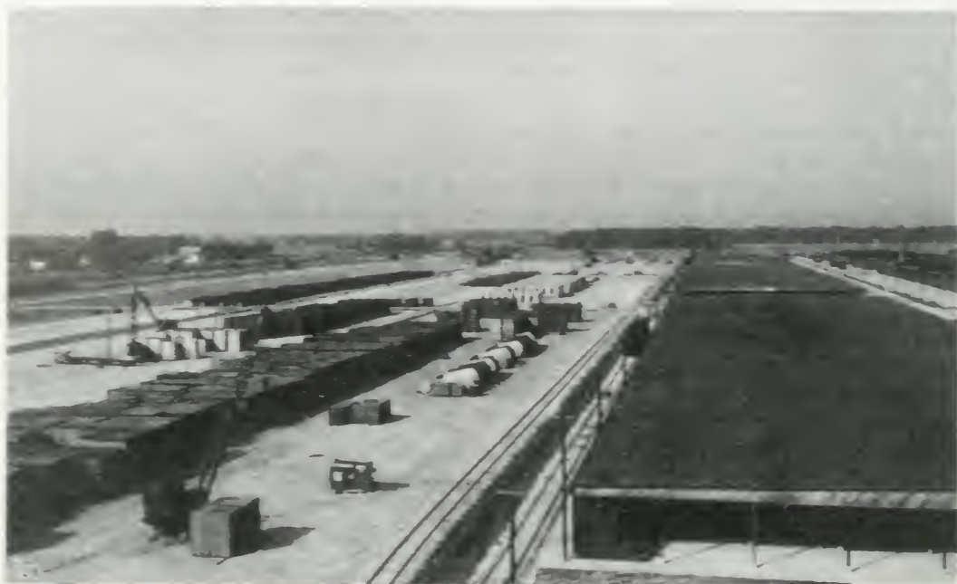
OPEN-TYPE STORAGE SHEDS (right) at Casad Ordnance Depot, New Haven, Ind., September 1943.
