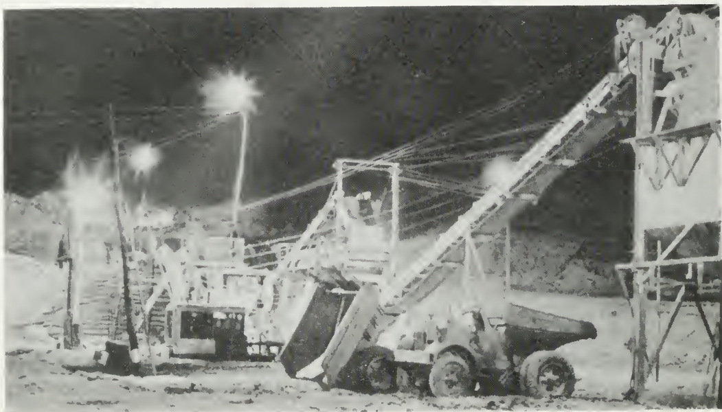
NIGHT CONSTRUCTION OPERATIONS in 1941 at Weldon Spring Ordnance Works, built for manufacture of high explosives.
