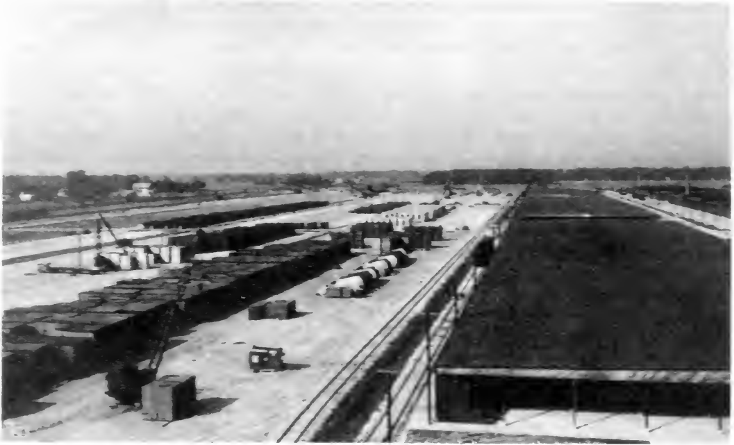
OPEN-TYPE STORAGE SHEDS (right) at Casad Ordnance Depot, New Haven, Ind., September 1945.
