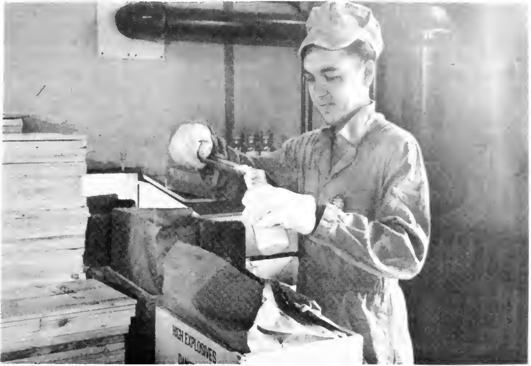
INSPECTOR AT VOLUNTEER ORDNANCE WORKS taking a sample of TNT for testing at an ordnance laboratory.
