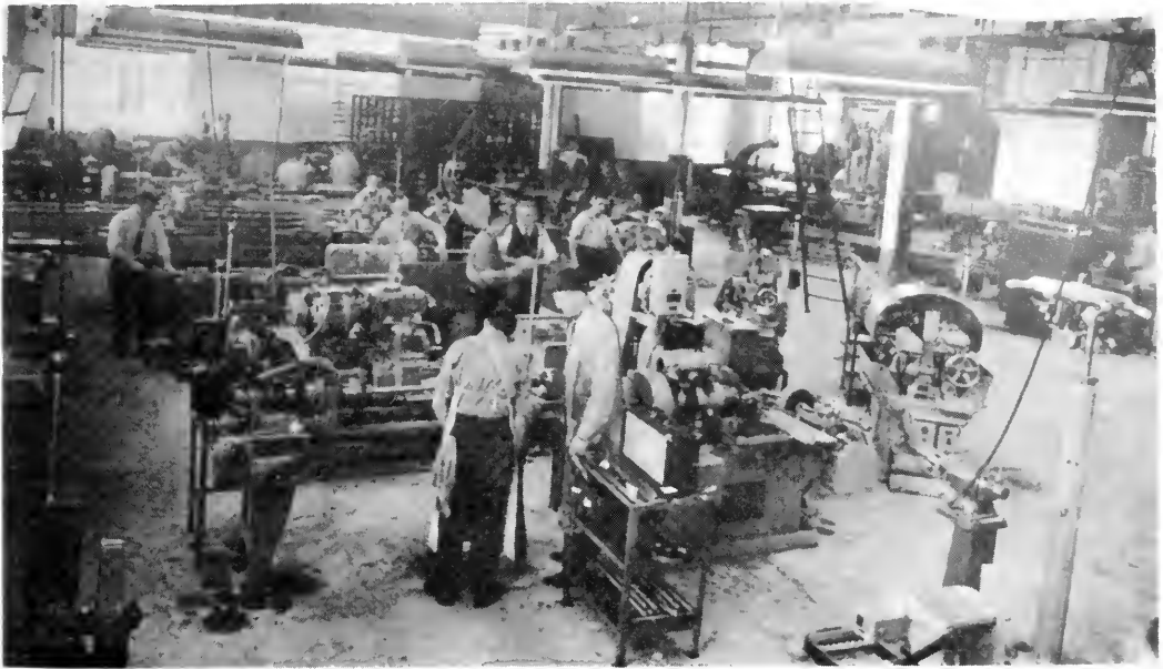
SAGINAW GUN PLANT, Mich., where machinery and equipment installed for operations on .30-caliber machine gun barrels are shown.
