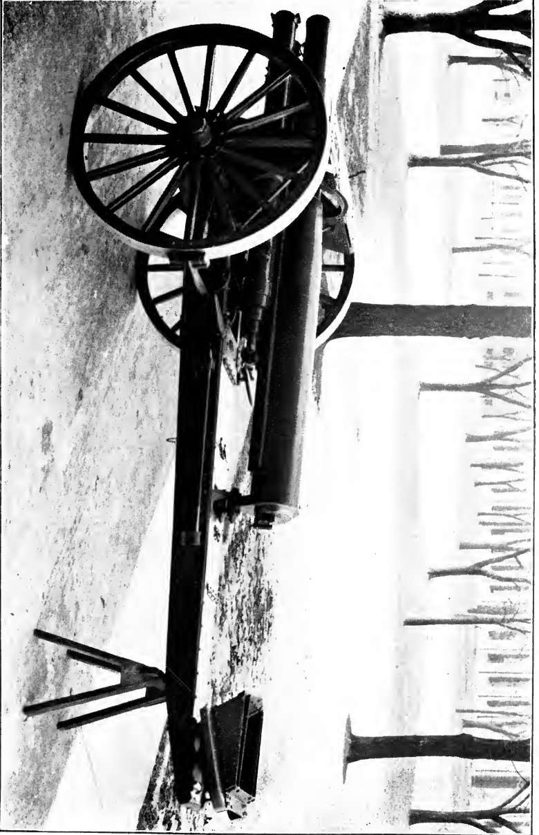
FIG. 129.—4.7-inch Siege Gun, Traveling Position.
