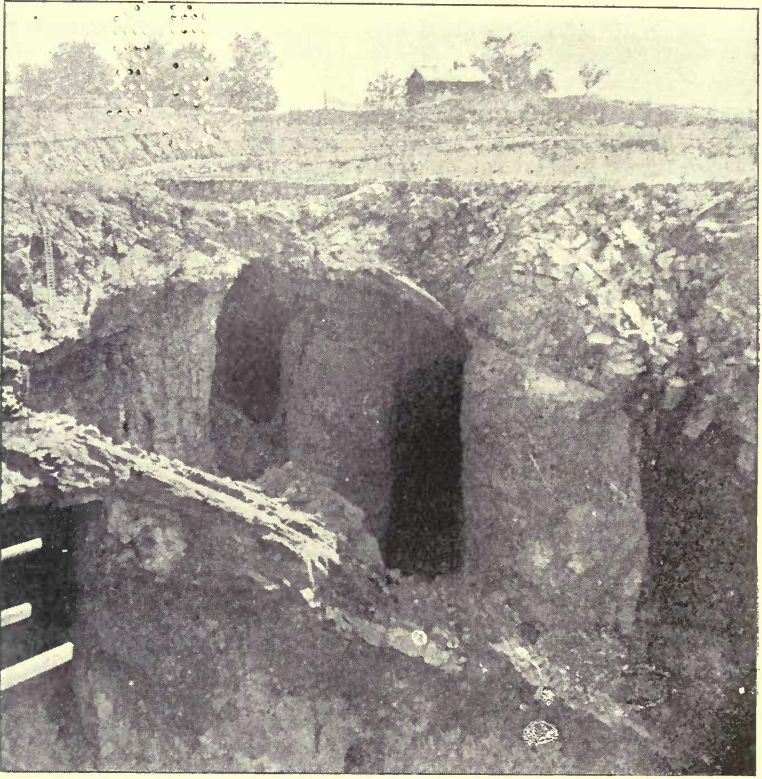
FIG. 46.—View of open cut and underground work in Mine 21, Mineville, near Port Henry, N. Y. Photographed by J. F. Kemp, 1892
