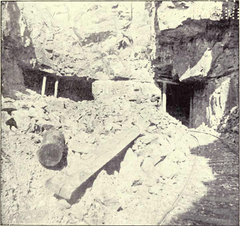
FIG. 43.—View of open cut at Pilot Knob, Mo., showing the bedded character of the iron ore. From a photograph by J. F. Kemp, 1888.
