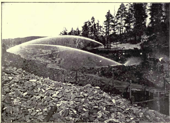
FIG. 137.—The Stevens Hydraulic placer mine, Auro City, Colorado. From a photograph.
