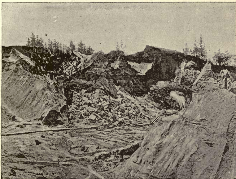
FIG. 59.—View of the Union diggings, Columbia Hill, Nevada County, California. From a photograph.
