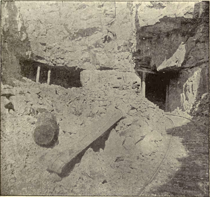
FIG. 23.—View of open cut at Pilot Knob, Mo., showing the bedded character of the iron ore. From a photograph by J. F. Kemp, 1888.
