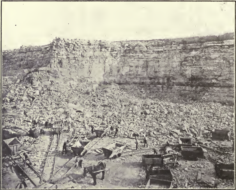
FIG. 79. — Quarry Showing Result of Blast.
