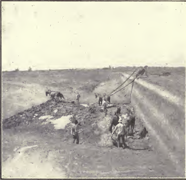
FIG. 80.— Stripping Coal by Scrapers.
