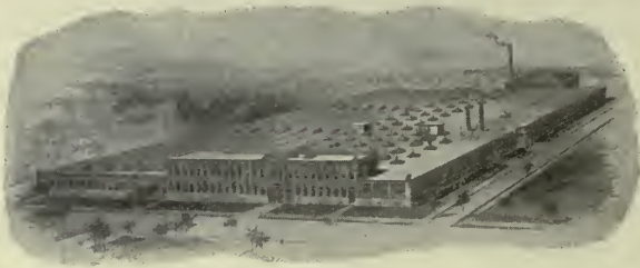
FIG. 25.—Factory of Potter & Johnson Co., Pawtucket, R. I., showing administration front, saw-tooth shop, and power plant, all practically under one roof.
