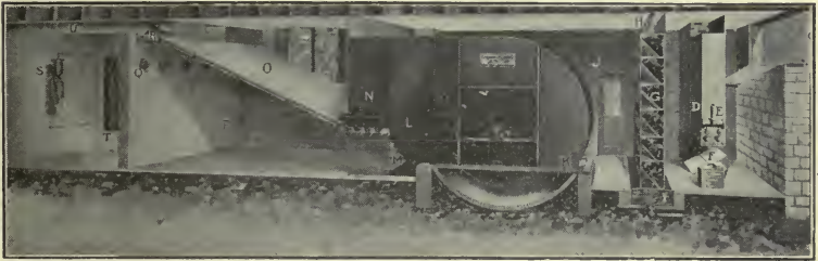
FIG. 22.—Hot-blast heater with coke air washer: C, screen through which outside air enters; D, tempering coil fed by steam pipe E; F, by-pass so air can go through without touching tempering coils; G, coke air filters moistened by perforated water pipe H; I, catch basin; K, blower; O, partition permitting part of the air to be blown over heater coils and part or all to be blown through ducts without passing over heater coils.
