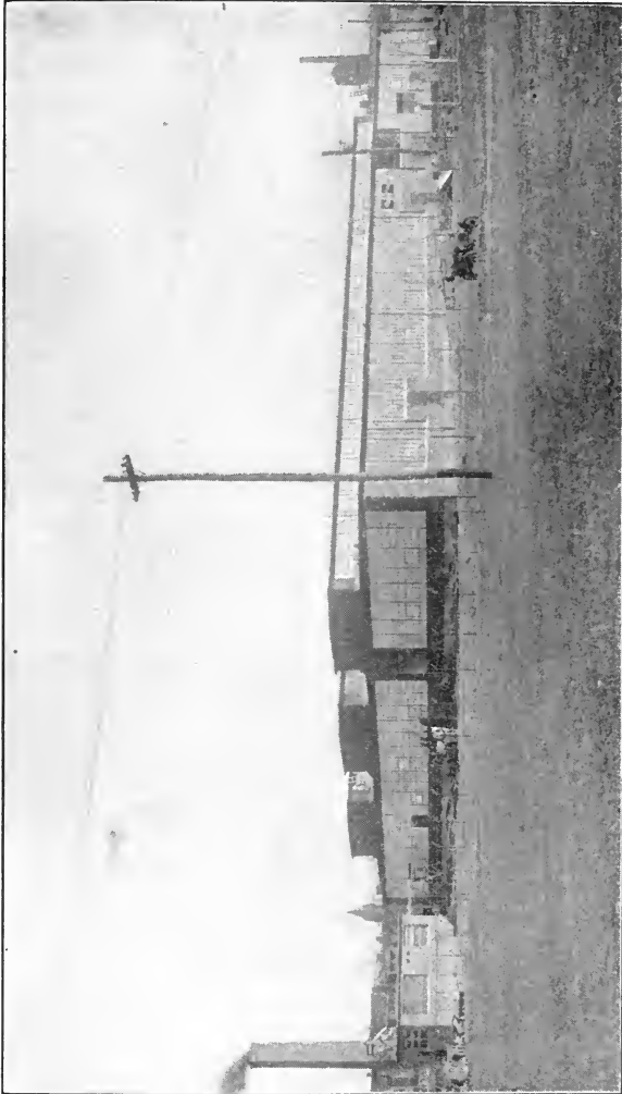
FIG. 20.—View of the factory of the Hero Manufacturing Co. Philadelphia, Pa. showing arrangement permitting expansion in all directions. Courtesy of the Austin Co., Cleveland, Ohio.
