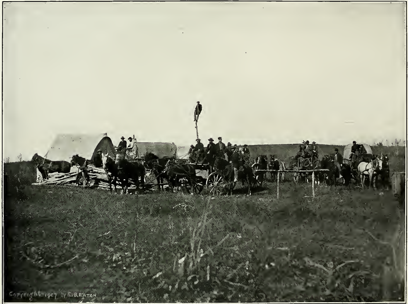
PHOTOGRAPH TAKEN AS MILITARY TELEGRAPH WAS BEING STRUNG
