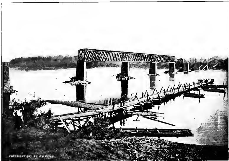
DESTROYED RAILROAD BRIDGE, BRIDGEPORT, ALABAMA—PONTOON IN COURSE OF CONSTRUCTION
