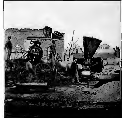
RUINED LOCOMOTIVE AFTER FALL OF RICHMOND IN 1865
