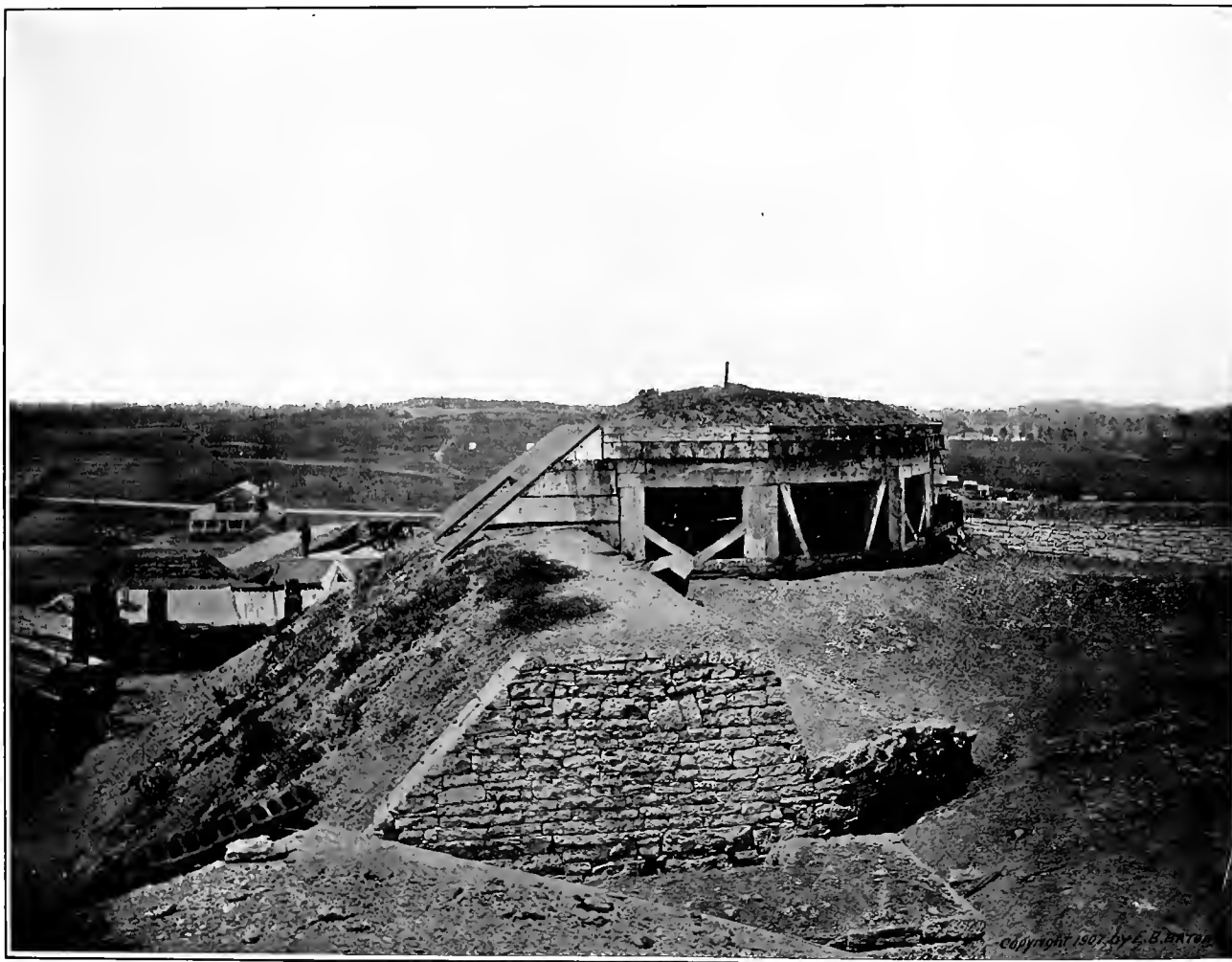
PHOTOGRAPH TAKEN IN FORT NEGLEY AT NASHVILLE, TENNESSEE, SHOWING IRONCLAD CASEMATES. IN 1864
