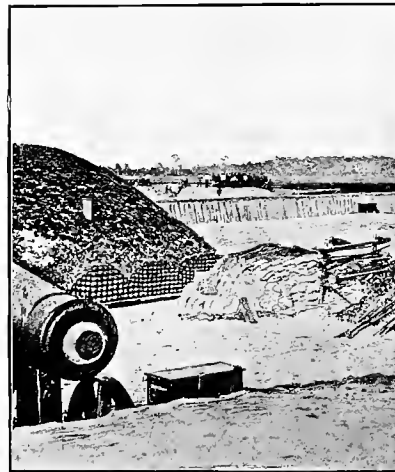
FORT BEAUREGARD, BAY POINT, S. C., 1861
