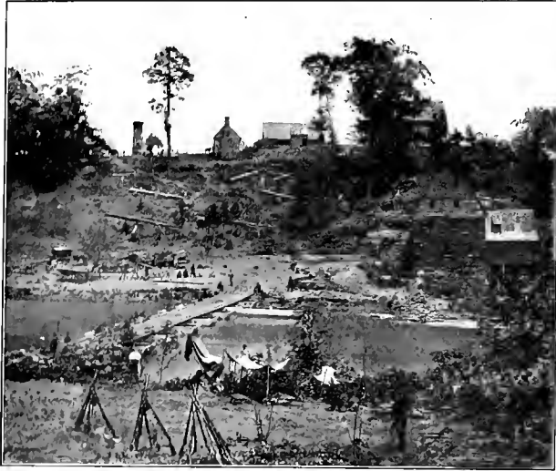
PONTOON BRIDGE AT JERICHO MILLS ON NORTH ANNA RIVER, VIRGINIA
