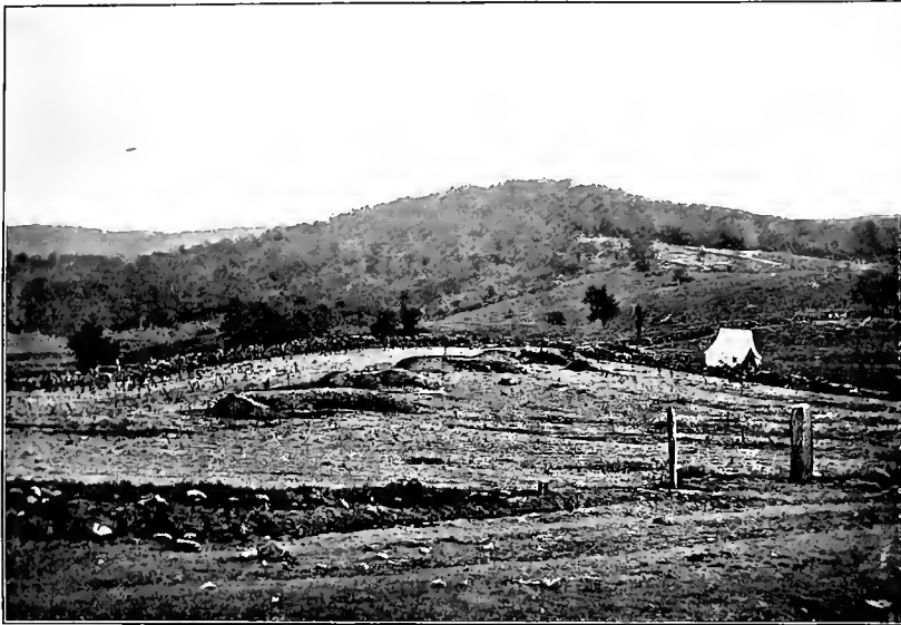
EARTHWORKS AT CULP'S HILL AT GETTYSBURG IN 1863
