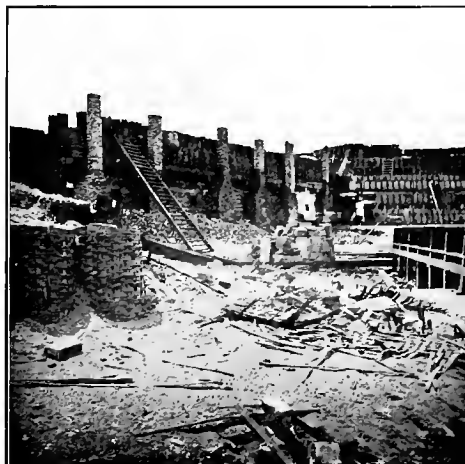
WRECKED INTERIOR OF FORT SUMTER
