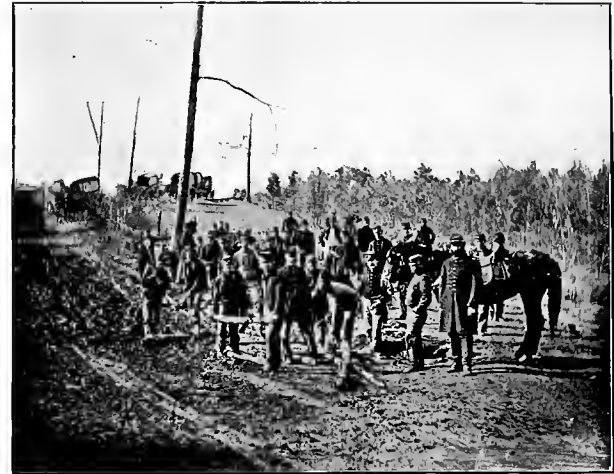
BUILDING A CORDUROY ROAD
