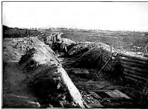
EARTHWORKS IN FRONT OF PETERSBURG—FEDERAL LINES AT FORT MORTON
