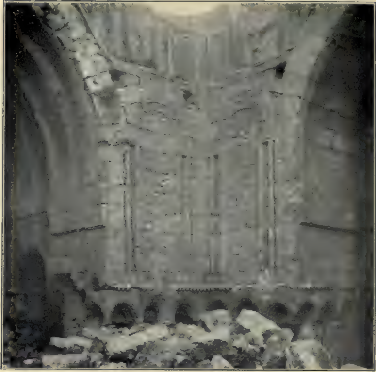
29 Ammān, square building with apse-buttresses ; blind arcade with formal ornament. See pp. 123, 124.
