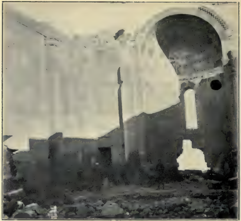
8 Ereruk, basilica with ruined barrel-vaults, and façade towers.
