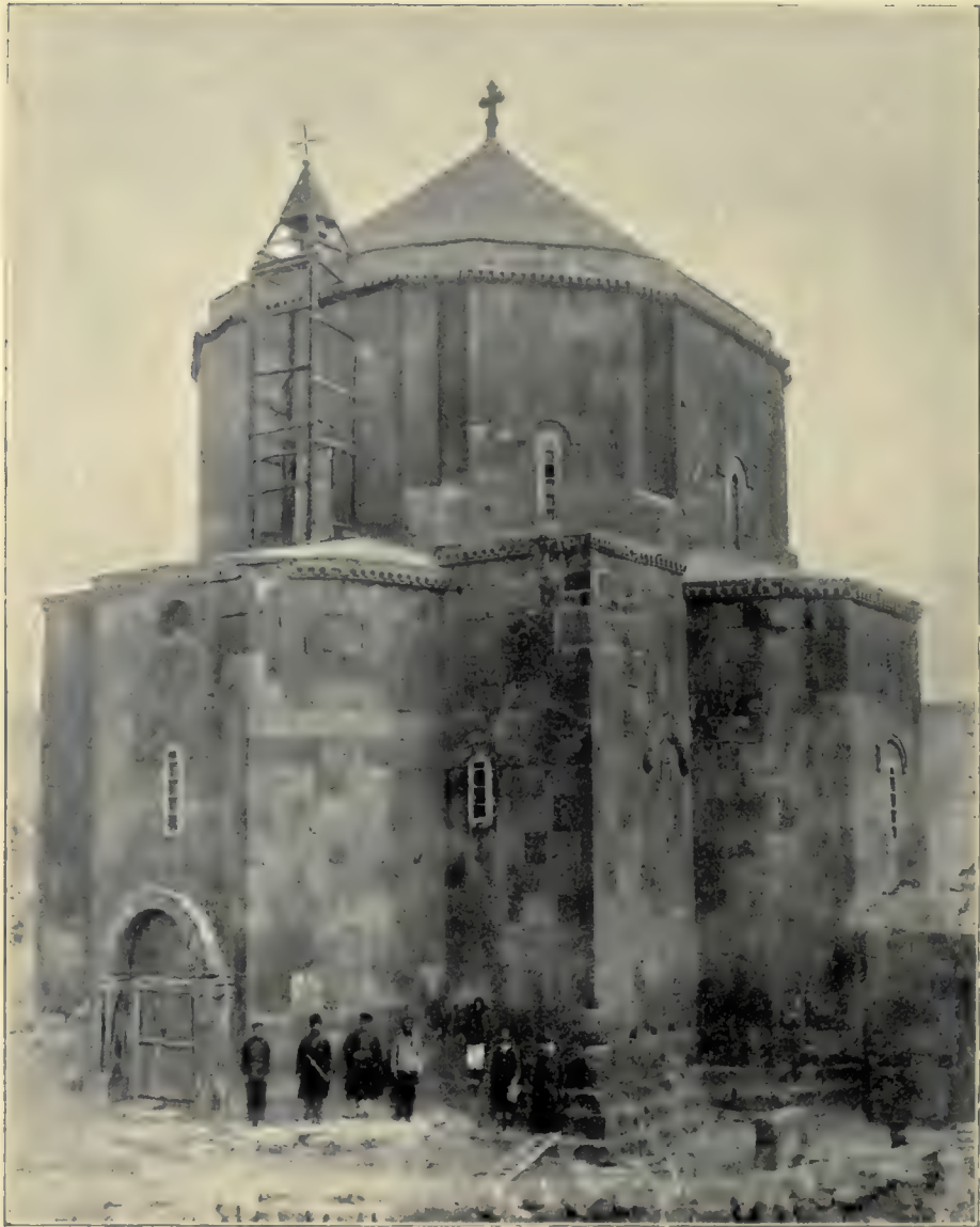
1 Maštara, domed square with apse-buttresses, c. A.D. 650 ; exterior from South-West. See p. 61.
