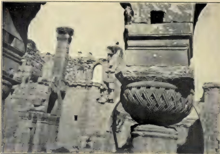
50 Meiafarqin, Church of the Virgin ; interior from West door ; photo., G. L. Bell. See p. 147.
