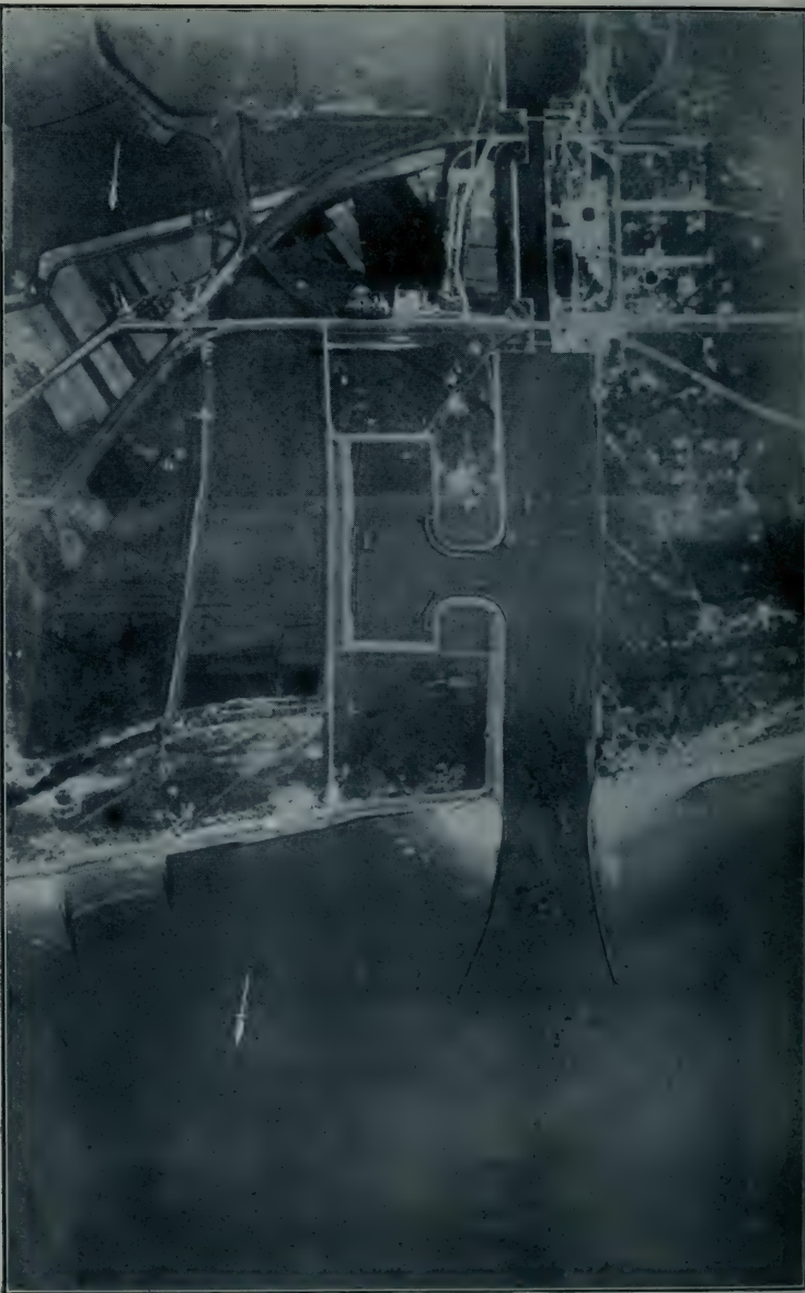
SEA-PLANE VIEW OF THE ZEEBRUGGE LOCK-GATES, SHOWING POSITIONS OF SUNKEN CRUISERS
