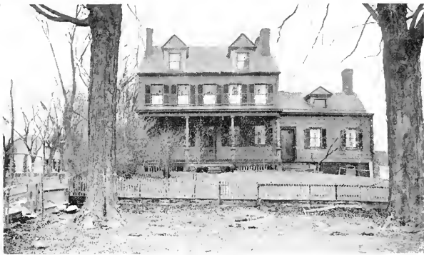
S. MERWIN MEAD HOMESTEAD Built 1809
