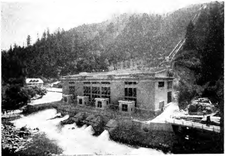
—Courtesy Pacific Gas and Electric Company. A power house in the high Sierras.
