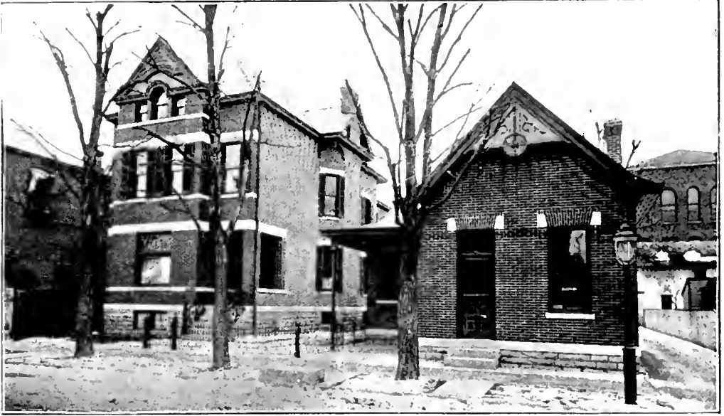
RESIDENCE AND OFFICE OF DR. H. A. COWING, S. High Street, Muncie.
